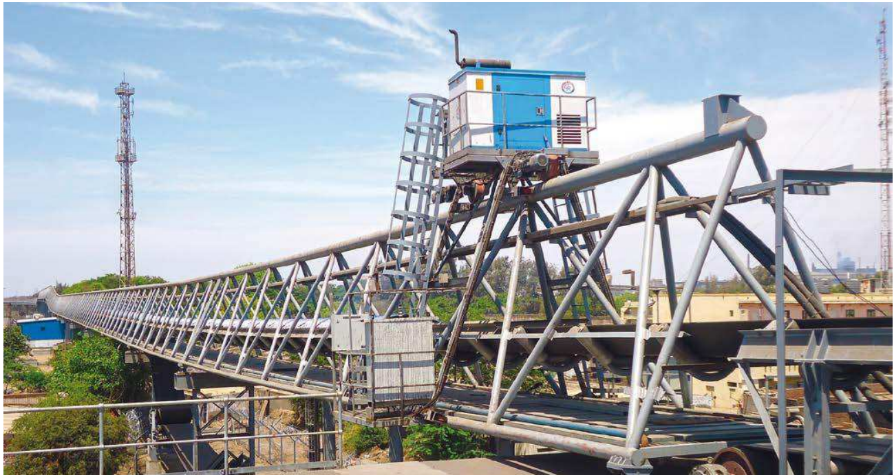
Pictures: © Conveyor Dynamics
